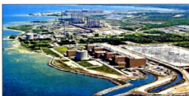
Bruce Nuclear Plant complex near Kincardine on Lake Huron, which houses eight separate reactors.
