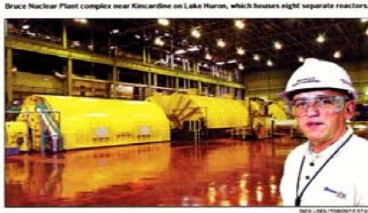
Duncan Hawthorne, chief executive of Bruce A, with Unit 4 ready for start up in the background.
