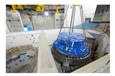
Fig. 2: The closure head of the Olkiluoto 3 reactor pressure vessel
