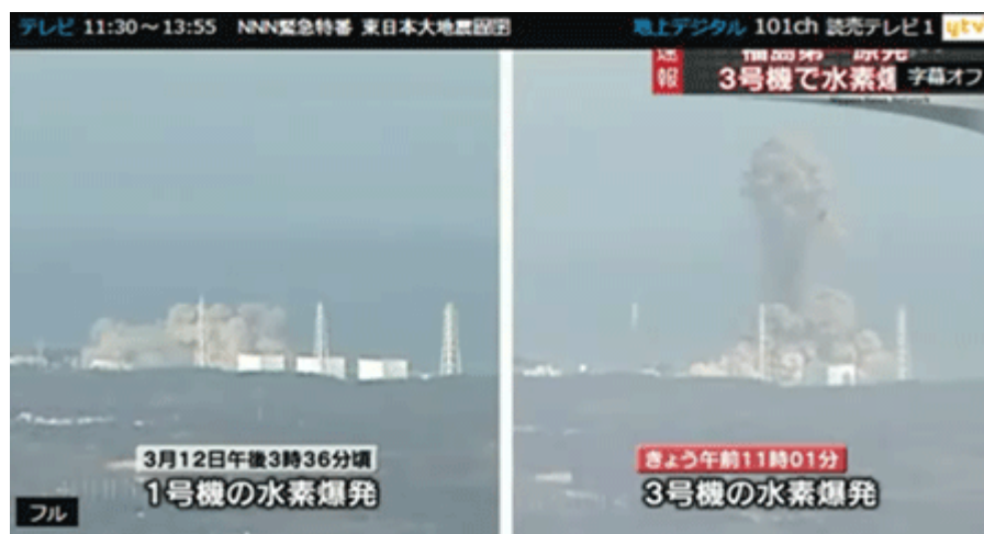
Figure 3: Hydrogen explosion at the Fukushima power plant
