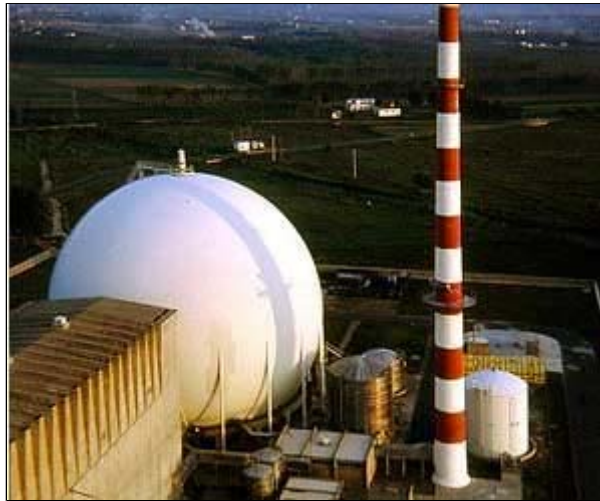
Garigliano nuclear power plant reactor building in 1970, to be decommissioned until 2016
