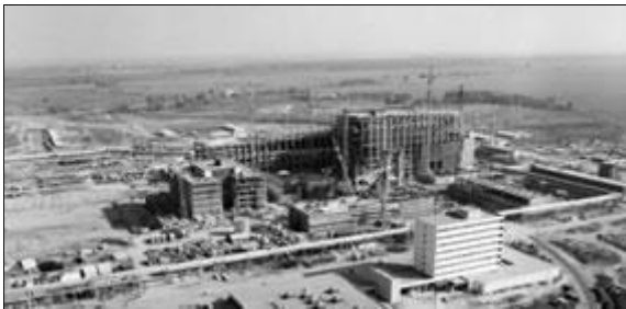
Fig.1. Constructions works at the Paks NPP
