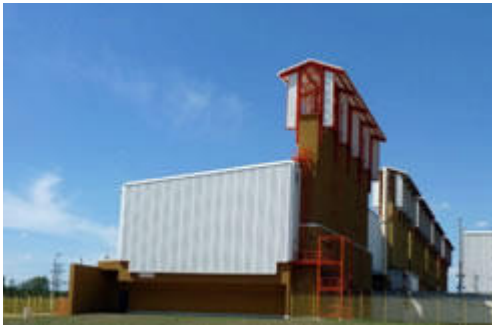
Fig. 3. Interim Spent Fuel Storage Facility
