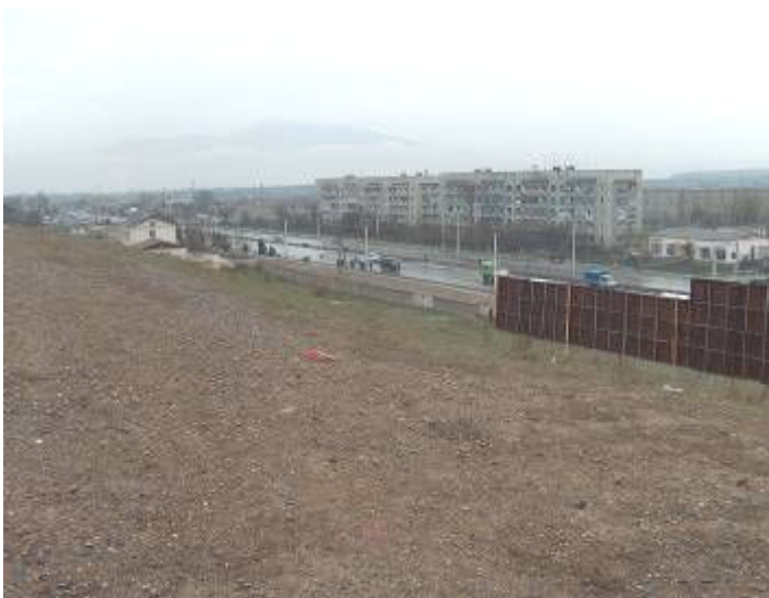
Fig. 1.2. Ghafourov tailings site: Note the proximity of dwellings, the cover appears intact with no obvious erosion features
