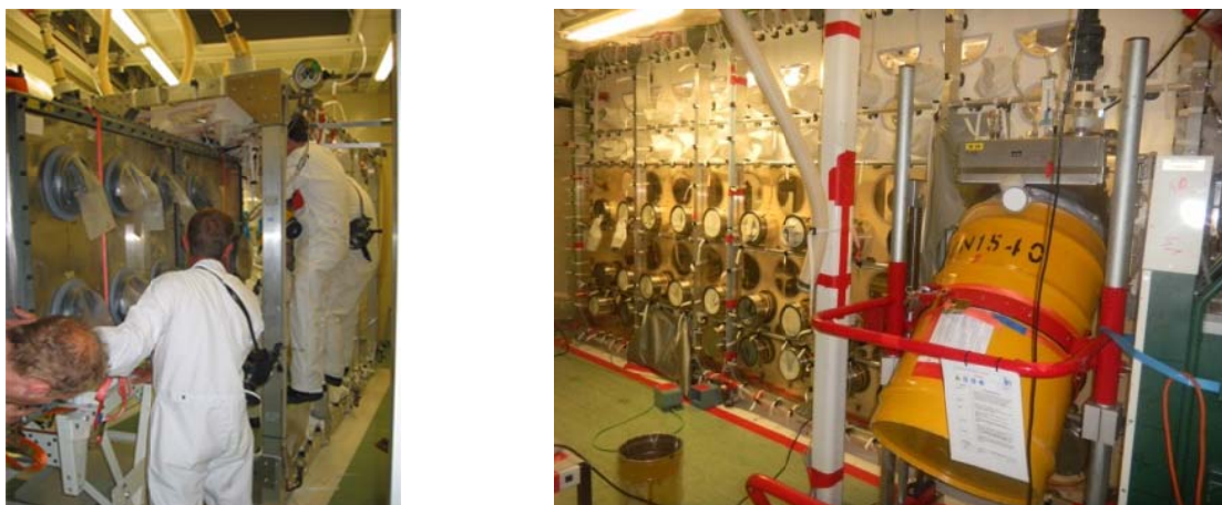
Figure 2: Typical dismantling tent with docking station
