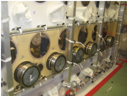
Figure 3: Modular shielding panels
