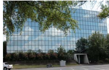
Figure 1 - Technical Training Center, Chattanooga, Tennessee
