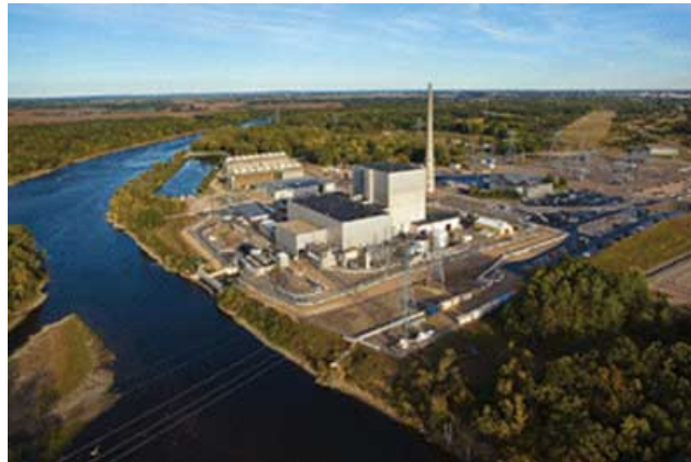
Fig 1: Monticello Nuclear Generating Plant
