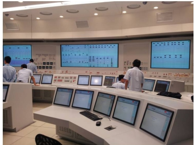
Fig. 2 Hybrid MCR: Fangjiashan NPP simulator (China)
