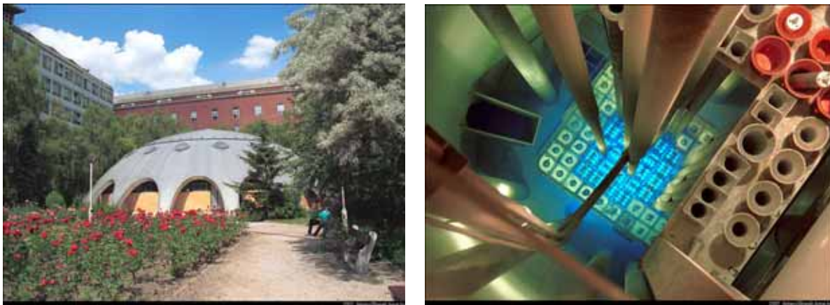
Figure 1. The reactor building and the reactor core at nominal 100 kW power
