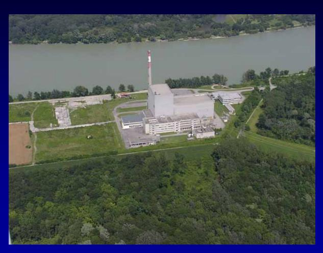
730 MW<sub>e</sub> Boiling Water Reactor (BWR Design model 69) built by KWU (originally AEG)
