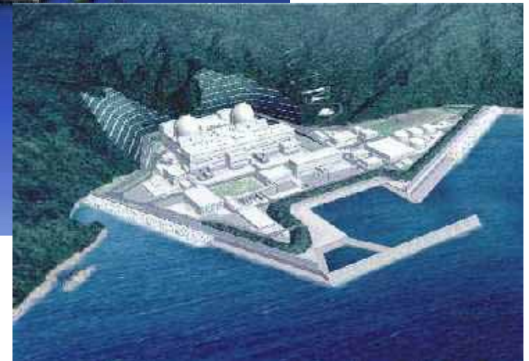
Tsuruga Plant No. 3, 4 (preparing for construction)
