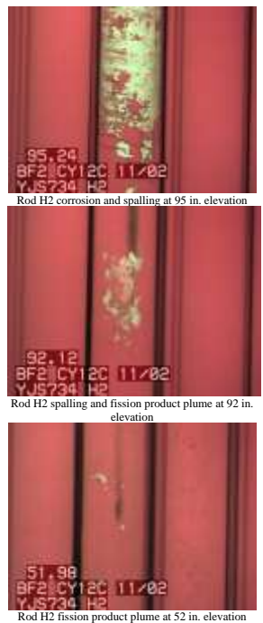
Figure 3: Visual Appearance of Failed BF-2 Reload 10 H2 Rod In Place in Bundle YJS734; Leaking Locations Near 52 and 92 inches and Heavy Spalling Starting Near 95 inches are Shown
