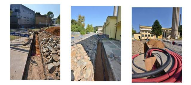
Fig.8 New electrical cables installation.
