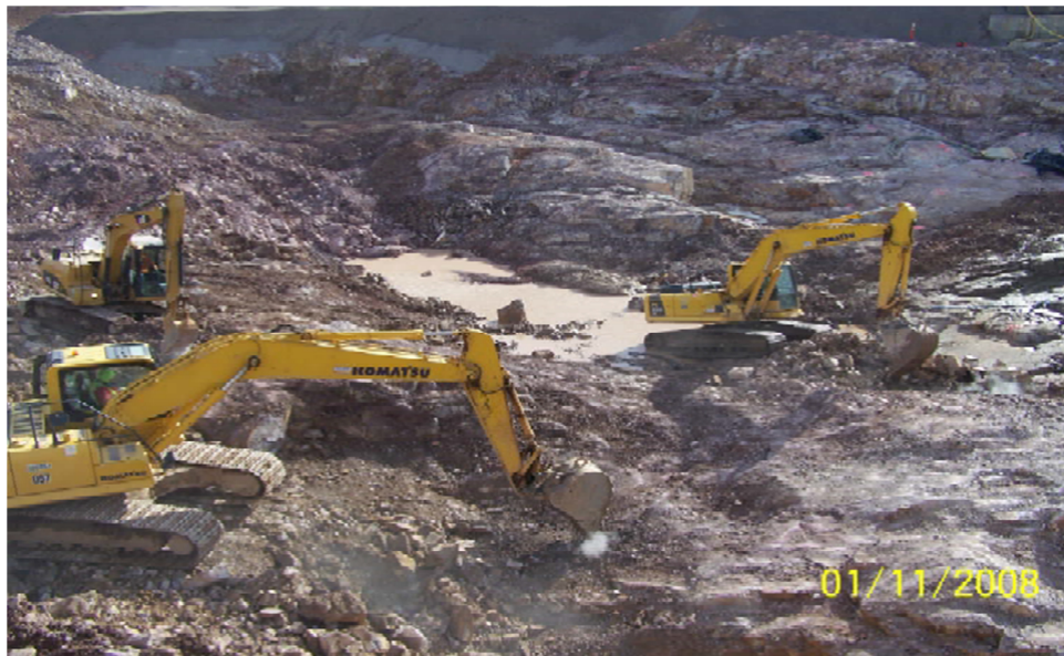
Fig. 1. Rock Clean-up prior to Dental Concrete and Leveling Concrete
