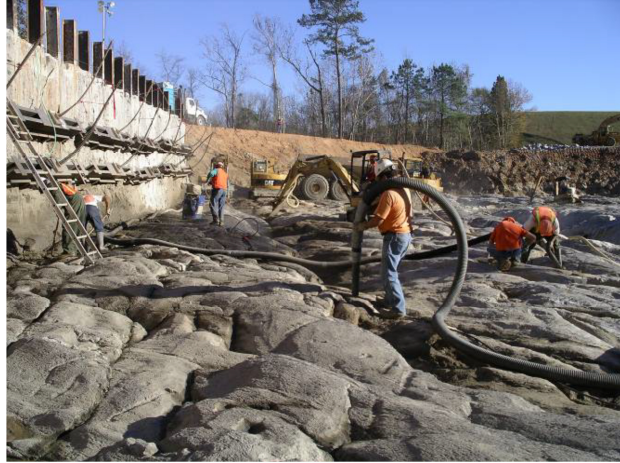
Fig. 2. Rock Preparation with Vacuum Trucks and Air Lances
