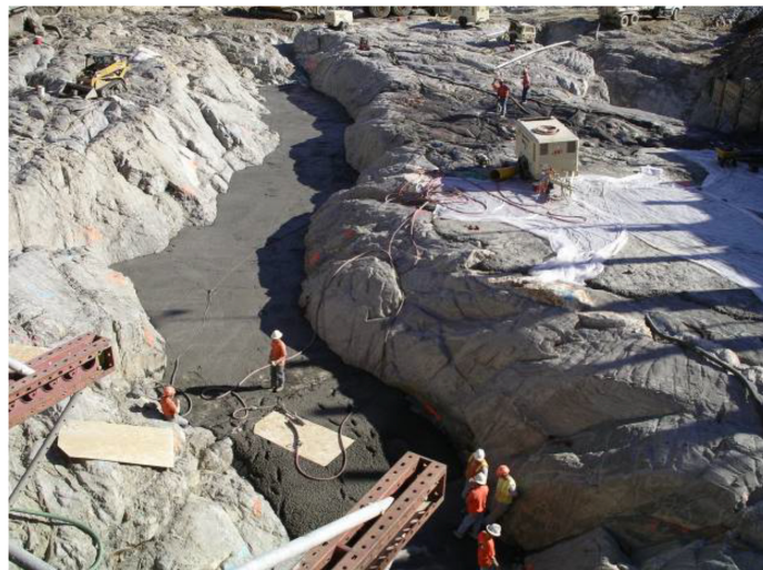
Fig. 3. Dental Concrete and Leveling Concrete Being Placed Adjacent a Mafic Dike
