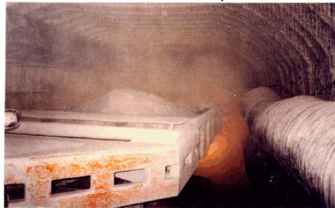
Backfilling Slinger Truck in a Disposal Drift
