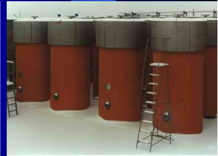
Existing SNF dry storage facility (capacity for 80 casks)
