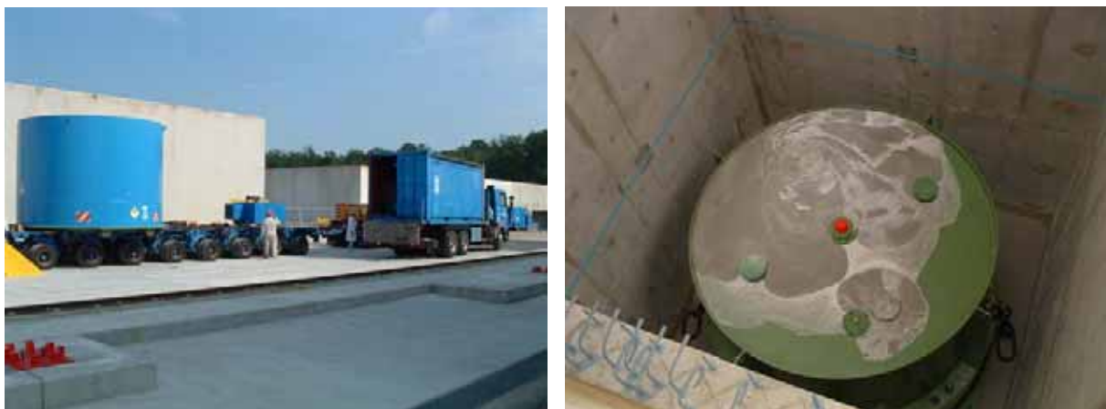
Figure 5: Transfer of a reactor-vessel cover towards the disposal-cell area ( left ) and placement in a disposal cell ( right ).
