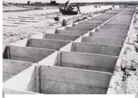
Figure 2: concrete disposal cells
