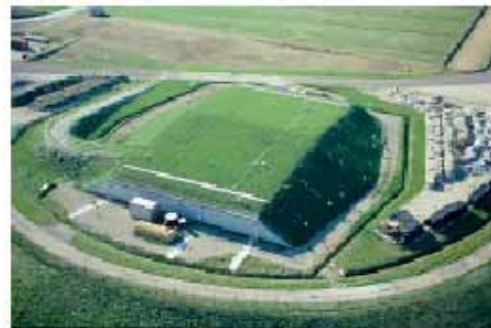
Figure 8: experimental capping system
