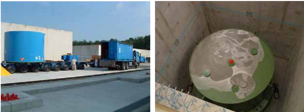
Figure 5: Transfer of a reactor-vessel cover towards the disposal-cell area ( left ) and placement in a disposal cell ( right ).
