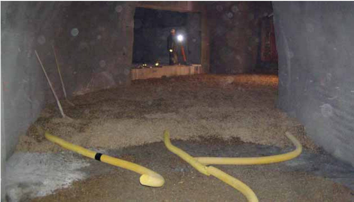
Picture 8: Construction of bottom drainage system
