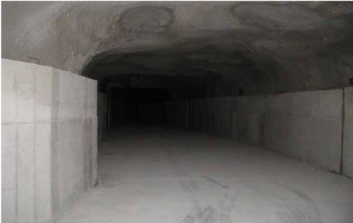
Picture 10: Completed part of the chamber 8/2
