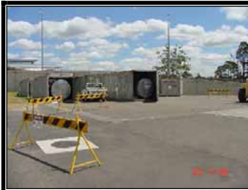
Cask Receipt/Inspection/Unloading Area
