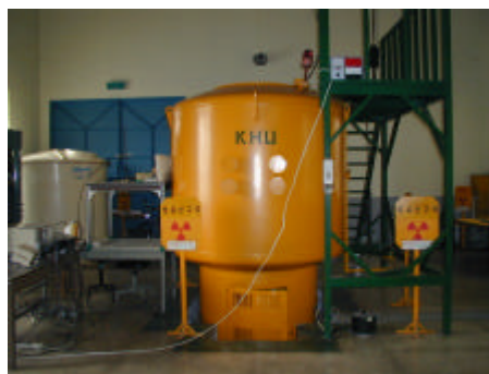
Fig. 1 Reactor Hall of AGN-201, KHU
