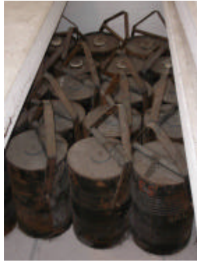
Fig. 1. Temporary storage of drums with EK-10 SNF in the HLWSF
