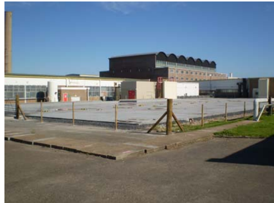
Photo 2 – Only Floor slab left
