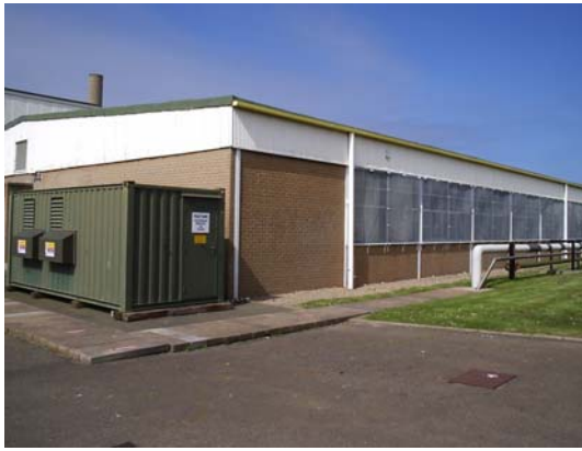
Photo 1 - D1202 before demolition commenced
