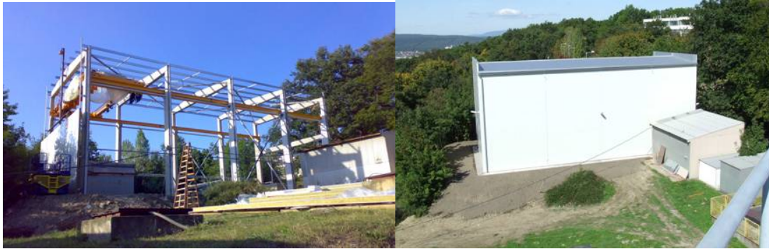
Fig.1. The transfer hall (left in construction, right ready)
