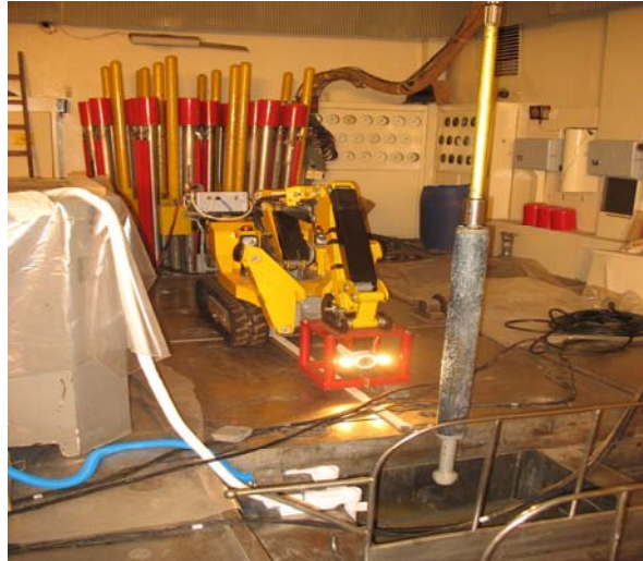
Fig.2. Radiation survey of the objects extracted from the sluice hatch.
