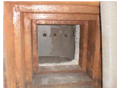
Fig 11. The TC after the dismantling
