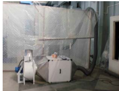
Fig 3. Temporary tent and ventilation
