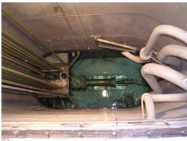
Fig 4. Reactor pool prior the dismantling
