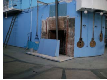
Fig 9. TC after the dismantling
