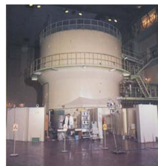
Fig 1. RA Reactor block
