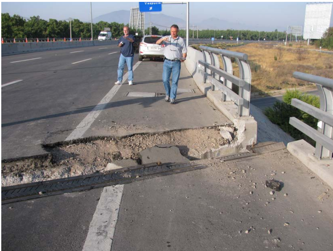
Fig. 1. Separation of the roadway.
