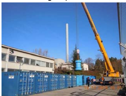
Fig 12. Loading SKODA casks into ISO-containers
