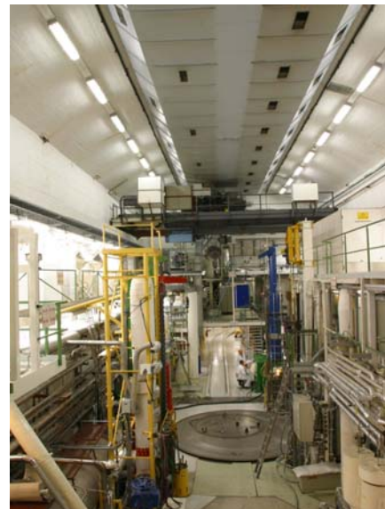
Figure 2 Halden reactor hall
