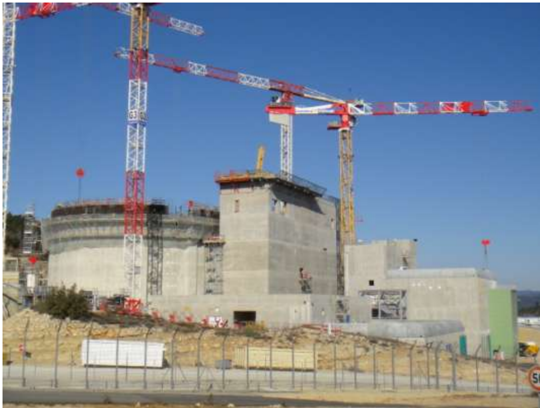
Figure 3 : View of the Building site march 2013
