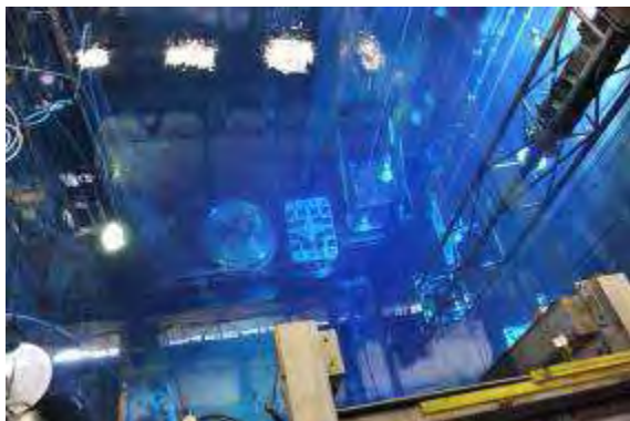
Fig. 15: The baskets used for RRSF transfer to wet storage © AREVA
