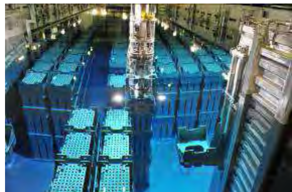
Fig. 16: RRSF storage-basket transfer to wet storage © AREVA
