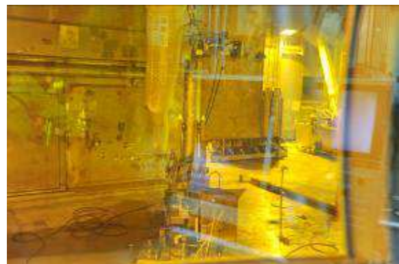
Fig.24: RRSF canister on top of the T1 dissolution pit © AREVA
