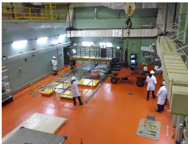
Fig. 5: View of the manoeuvres with the shielded container during the fuel discharge operations in order to position it on top of the auxiliary pool.
