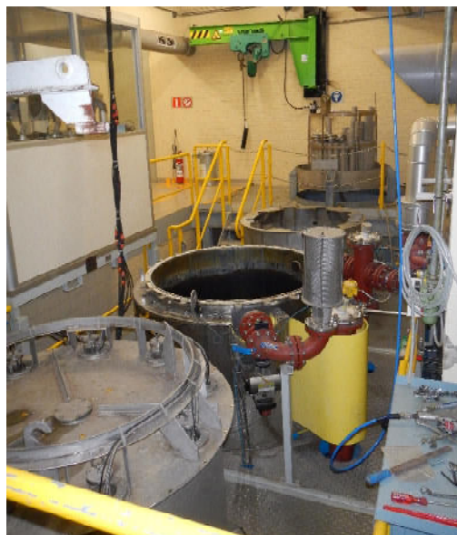
Figure 8: MEDOC® chemical decontamination workshop
