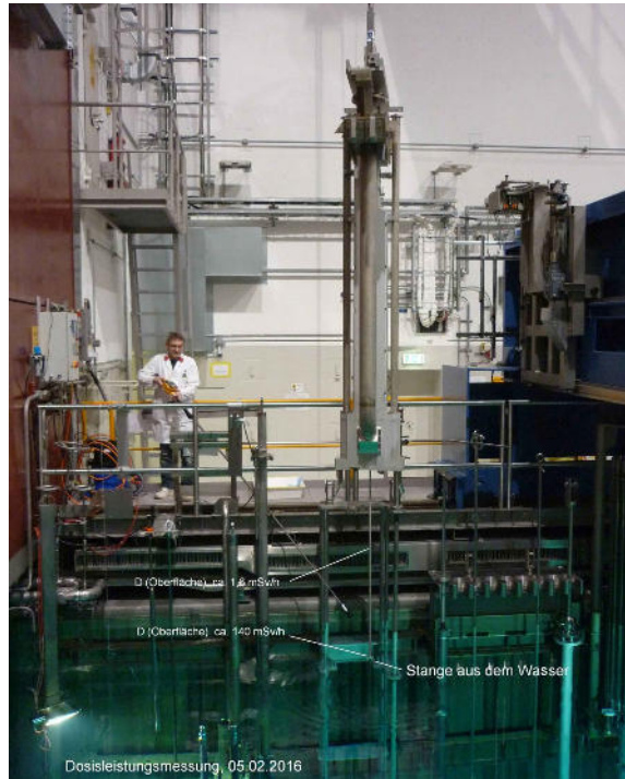
Fig 6. Checking the dose rate during pulling out of water of the outer duct
