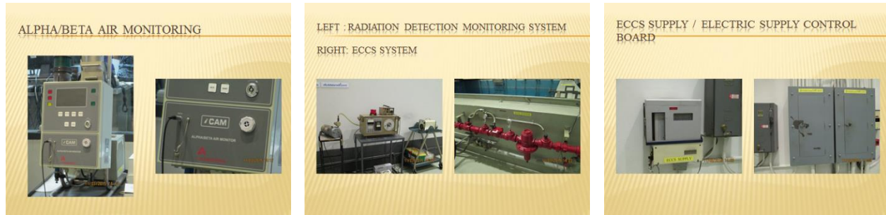
Fig. 3 Nuclear security practices of 2 MW TRR-1/M-1, TRIGA MARK III
