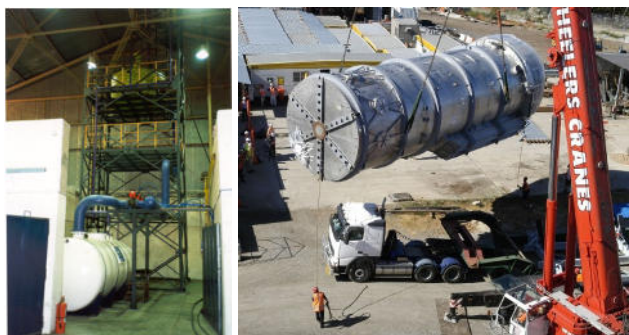
Figure 1: SSS mock up and transportation of the Reactor Pool
